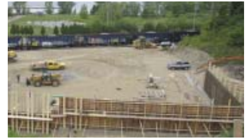
Construction begins for Waterfront Apartments
